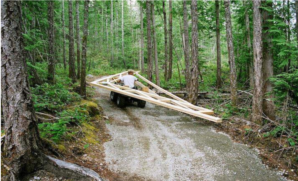
Figure 4 - Using the Quad to transport building materials
