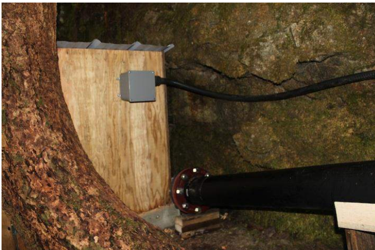
Figure 7 - Turbine house built on rock ledge and protected from washout by a tree.
