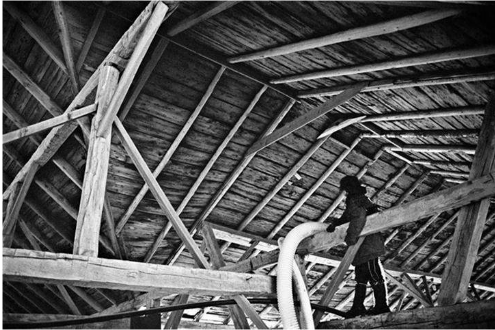
Kaye helps store extra building supplies in the rafters of the old barn during a community clean-up day.
