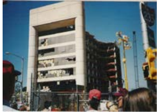
The Alfred P. Murrah Federal Building after being targeted by the Oklahoma City bombers.
